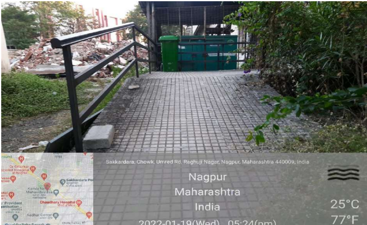
Ramp for physically Disabled person
