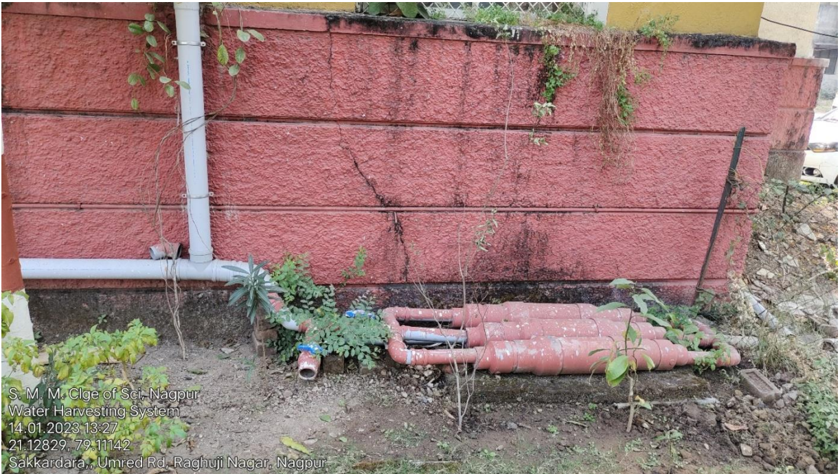
Arrangement of rain water harvesting system
