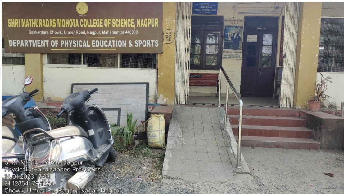
Ramp for PwD in front of Department of Physical Education and Sports
