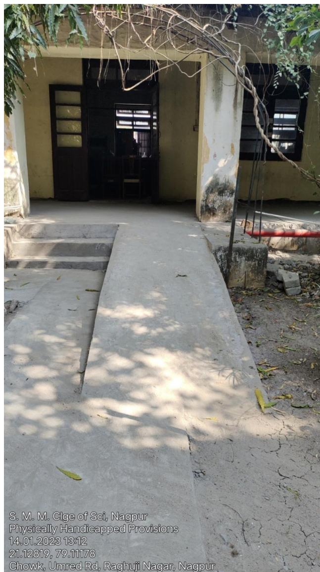
Ramp for PwD in front of Chemistry laboratory leading to the main office
