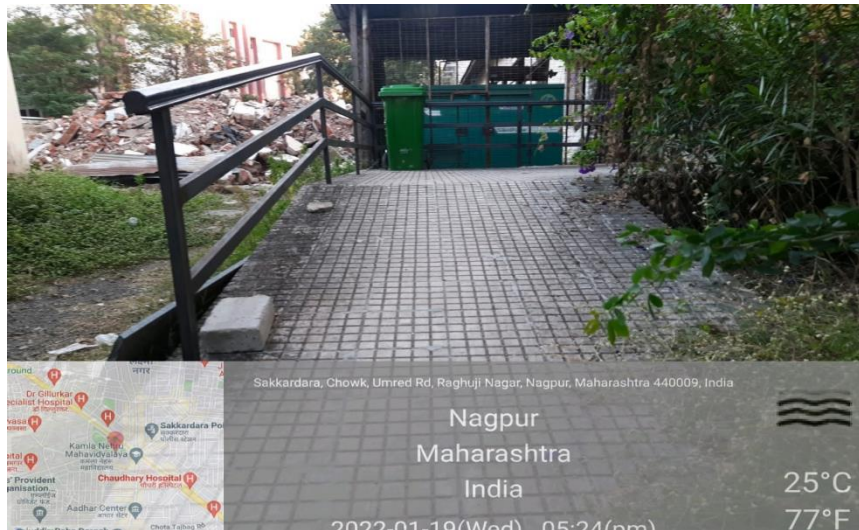
Ramp for PwD
