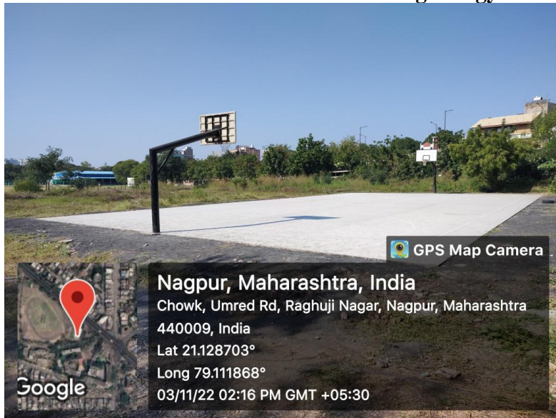
Newly constructed basketball court
