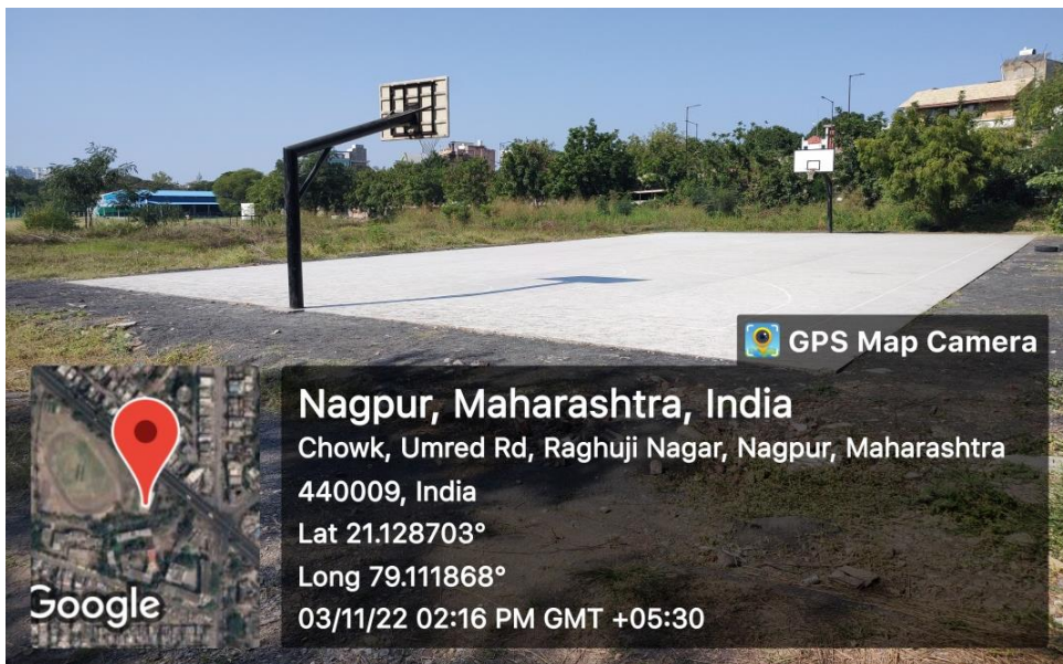
Newly constructed basketball court
