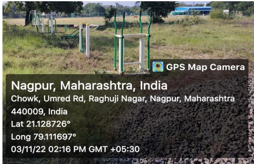
Installation of green gym in the college
